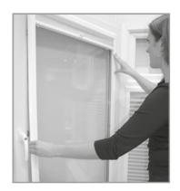
To ensure all brackets are in the correct position for fitting (85mm from beading) use a credit card in the corner of the window to locate the bracket position.
